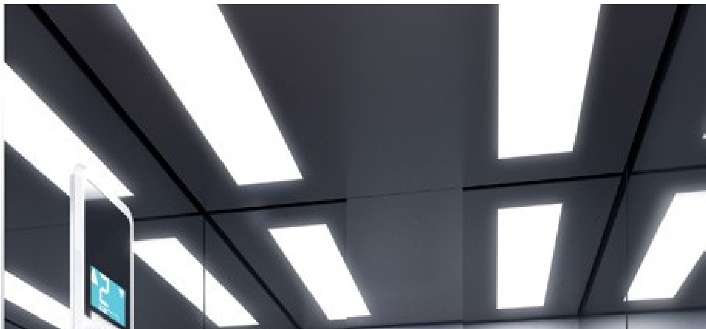
LINEAR LIGHT OVER A MIRROR CABIN – IN PLACE
